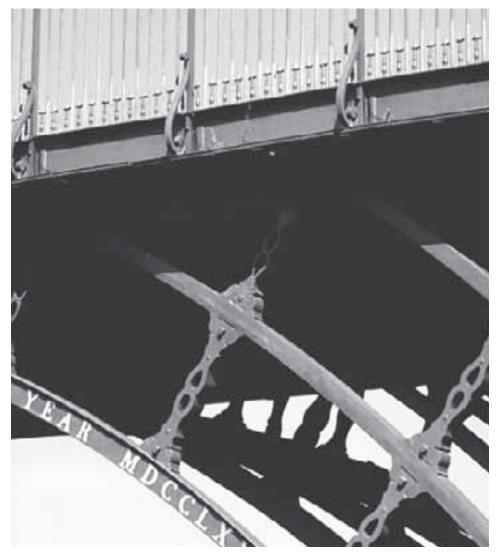
Figure C6 Joints in the bridge at Ironbridge
