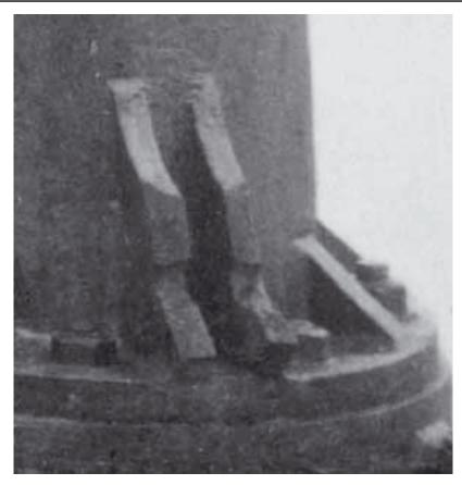
Figure C16 Fractured lug on pier 3
