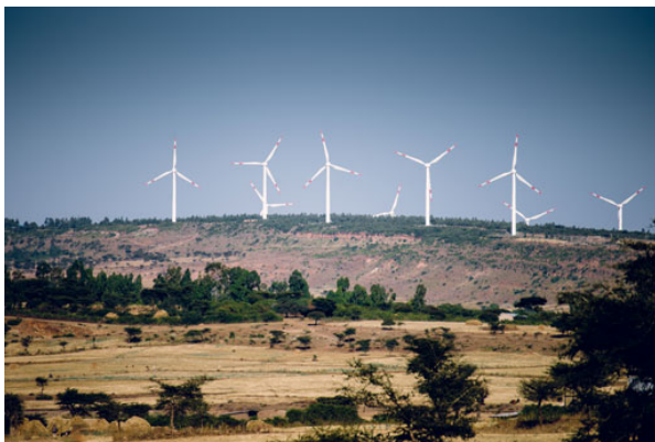
Figure 15.6 Wind farm near Adama producing renewable energy.
