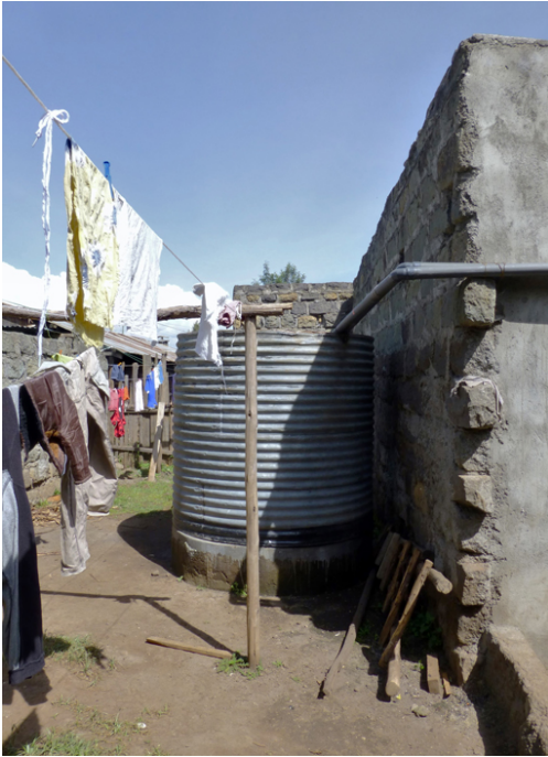
Figure 11.4 Rainwater harvesting tank collecting water from the roof of a housing block.
