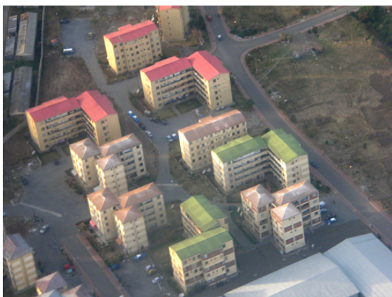
Figure 15.3 Aerial photo of condominiums on the outskirts of Addis Ababa.
