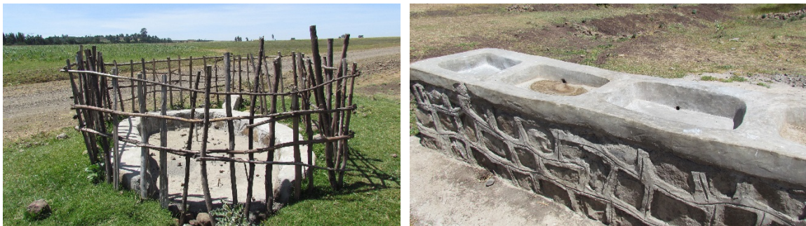
Figure 10.1 Debero-Garmojo water supply system showing (left) protected spring eye and (right) the cloth washing basin.
