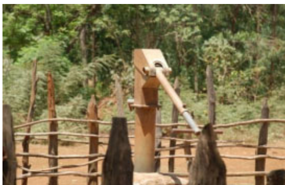
Figure 14.2 A non-functional hand-dug well. Only 2000 birr was needed to repair the pump.
