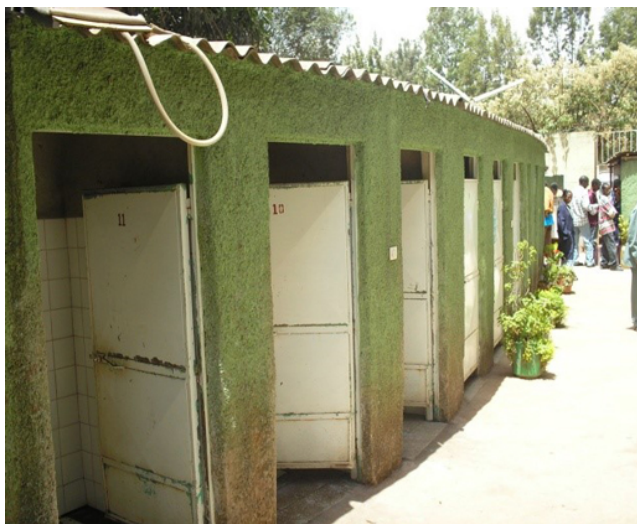
Figure 14.3 A public latrine block in Addis Ababa.
