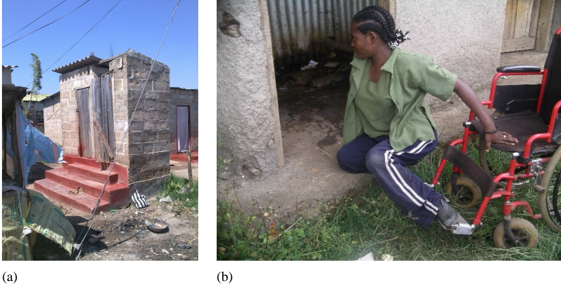
Figure 8.7 The different needs of people with disabilities must be considered when planning and building latrines.
