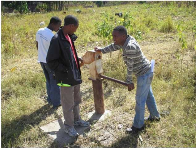
Figure 6.1 A hand pump – abandoned because it no longer works.
