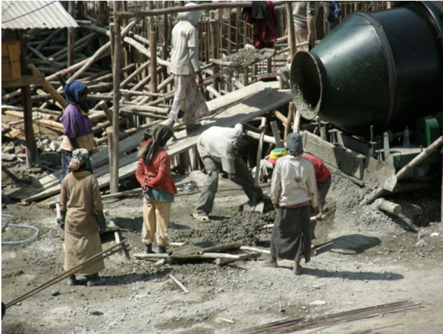
Figure 6.2 Construction of new buildings uses many different resources.
