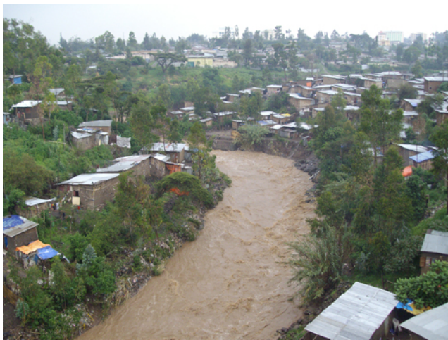
Figure 2.8 Informal dwellings built close to the Akaki River in Addis Ababa are vulnerable to flooding.
