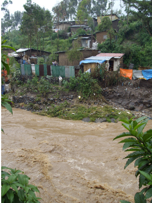
Figure 6.4 Houses perched precariously close to the flooding Akaki River in central Addis Ababa.
