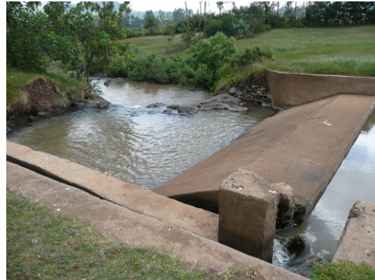
Figure 4.6 Small dams hold back river water so it flows into irrigation channels.
