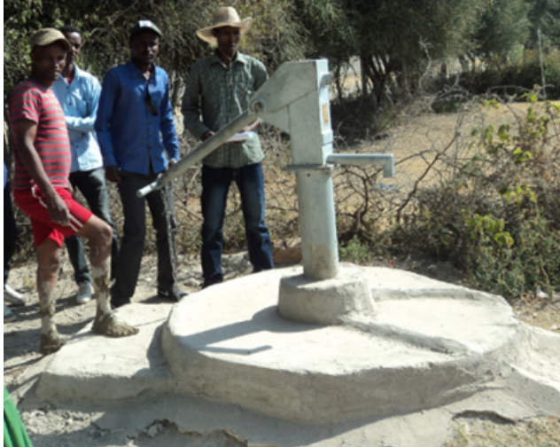
Figure 15.4 A newly constructed hand pump.
