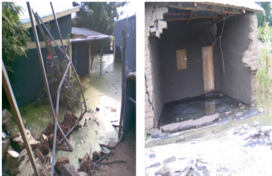
Figure 10.1 Homes damaged by the 2006 flood in Gambela town, Ethiopia.
