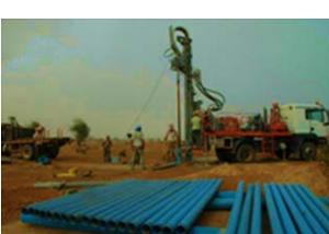
Figure 3.8 Drilling rig for a borehole.
