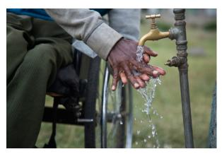
Figure 9.2 Water taps must be placed so that they are accessible to everyone.
