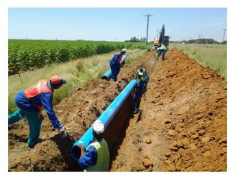
Figure 7.2 Plastic water mains being laid.
