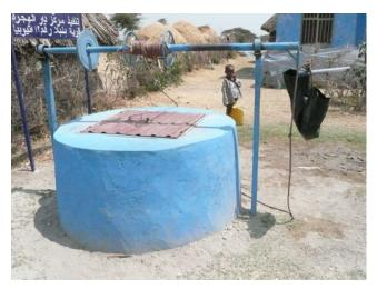
*Figure 3.5 Protected well with concrete surround and a lid. Note the black plastic bucket is suspended off the ground to keep it clean.*
