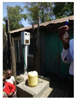
*Figure 13.5* A prepaid water meter. The man standing to the right is holding the small blue credit token that is inserted into the meter to obtain water.
