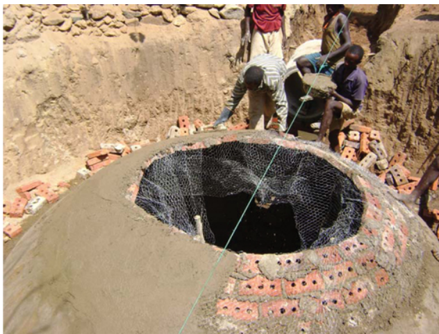
Figure 13.3 Biogas digester under construction.
