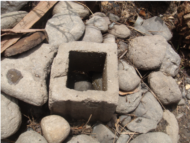
Figure 6.16 Pit for disposal of sullage
