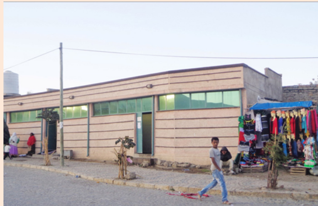
Figure 13.1 This public latrine was developed as a commercial opportunity for women in Mekelle town, Tigray region.
