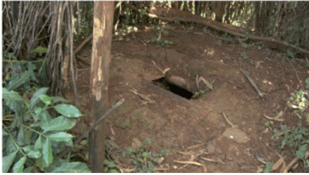
Figure 5.2 Traditional pit latrine with no slab.
