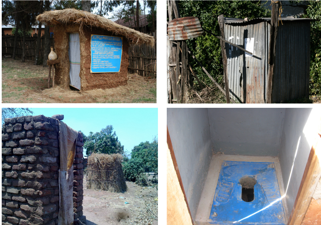
Figure 5.7 Pit latrine superstructures made of different materials.
