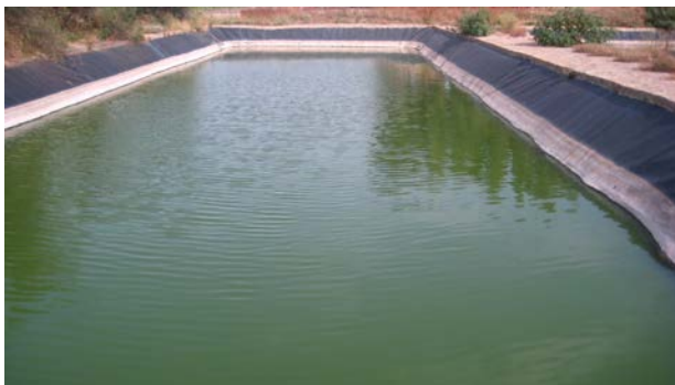
Figure 6.10 A waste stabilisation pond at Mekelle University – note the green colour of the pond due to algae.
