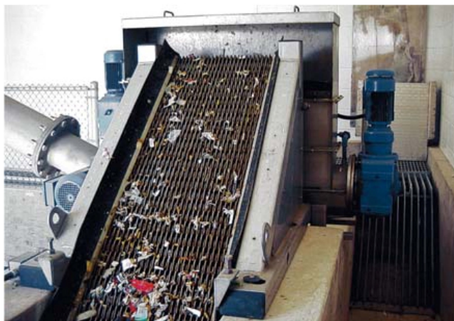
Figure 6.13 Screening of wastewater. Solid materials are retained on the screen while the liquid passes through.
