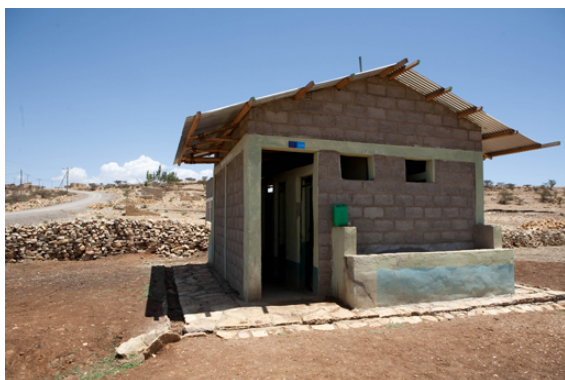
Figure 12.2 New school latrine block with handwashing facilities.
