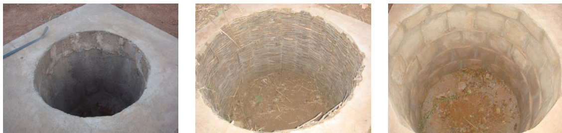
Figure 5.8 Pit linings made from stones, bamboo and blocks.
