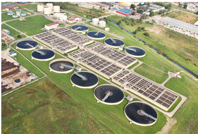
Figure 6.12 A mechanical-biological wastewater treatment plant.
