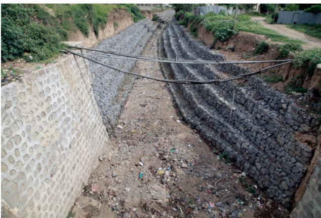
Figure 6.17 Stormwater drain designed to prevent flooding in Adama.
