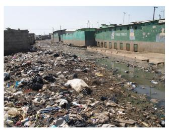
Figure 1.4 Accumulated solid waste and effluent from a latrine block have filled a drainage canal in Accra, Ghana.
