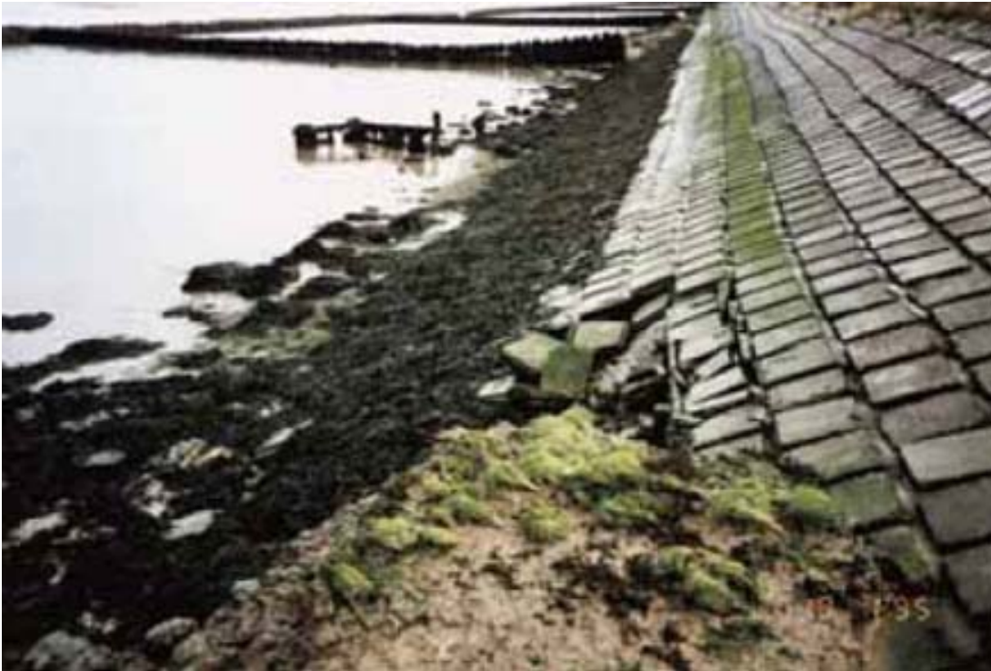
Figure 7 Reinforced sea walls.
