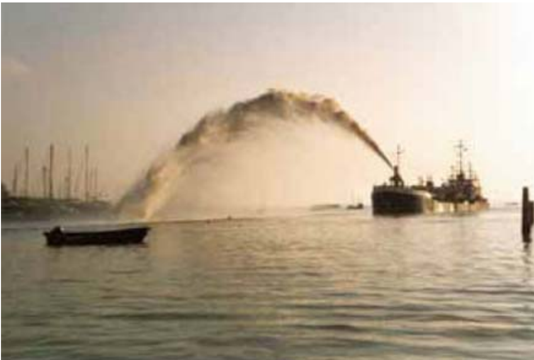
Figure 6 Recharging protects the coast by creating offshore barriers.
