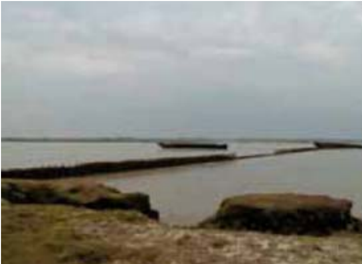
Figure 18 Sunken lighters help to defend the coast against wave action.
