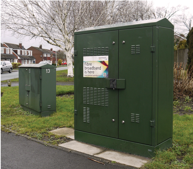
Figure 25 Fibre box used with VDSL2
