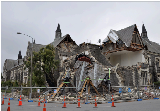
Figure 6 Earthquake in Christchurch, New Zealand
