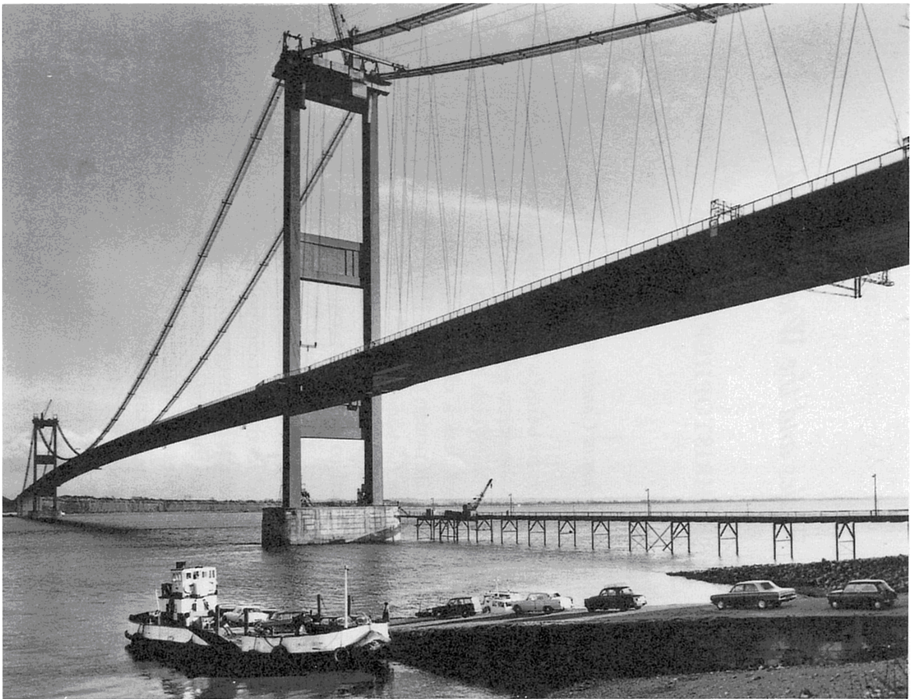
Constructing the Severn Bridge, c.1965
