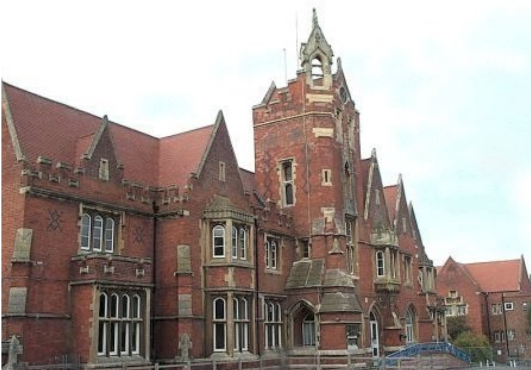
Figure 12 Warley Hospital in Essex was an old asylum closed at the start of the twenty-first century.
