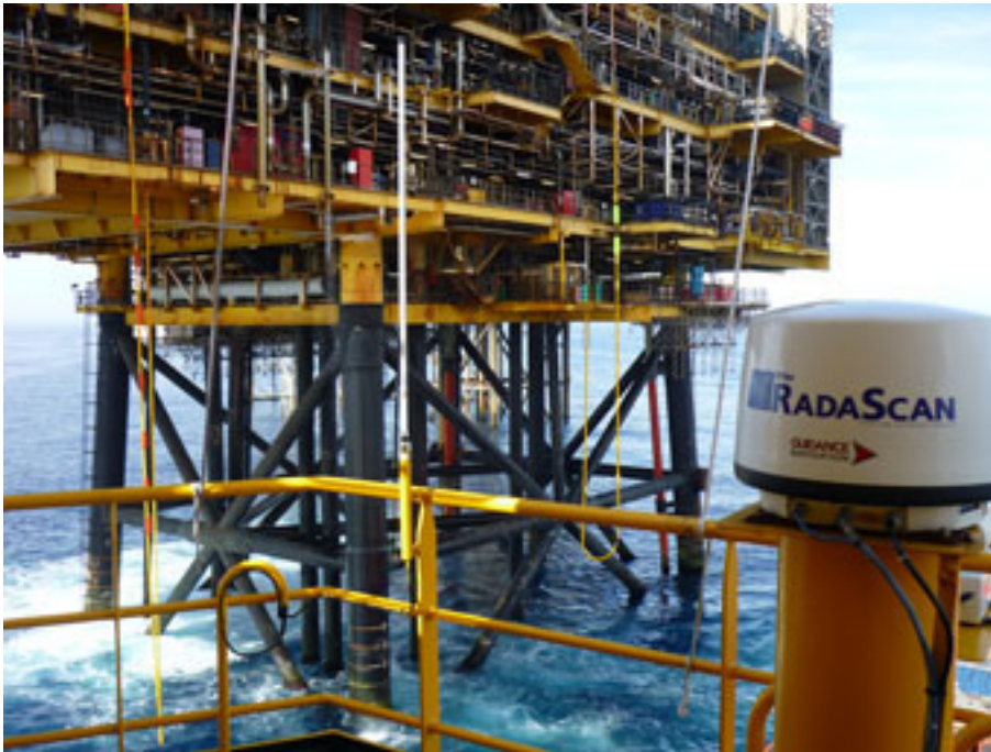
Figure 8 A Guidance radar sensor at work
