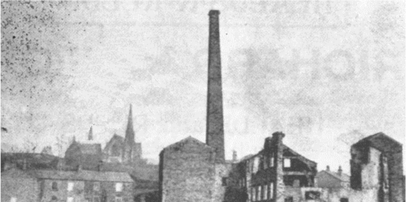
Aitkens and Lords Mill, Chatterton, before demolition in 1890s.
