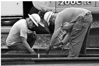
Figure 1 Engineering work carried out on a rail track
