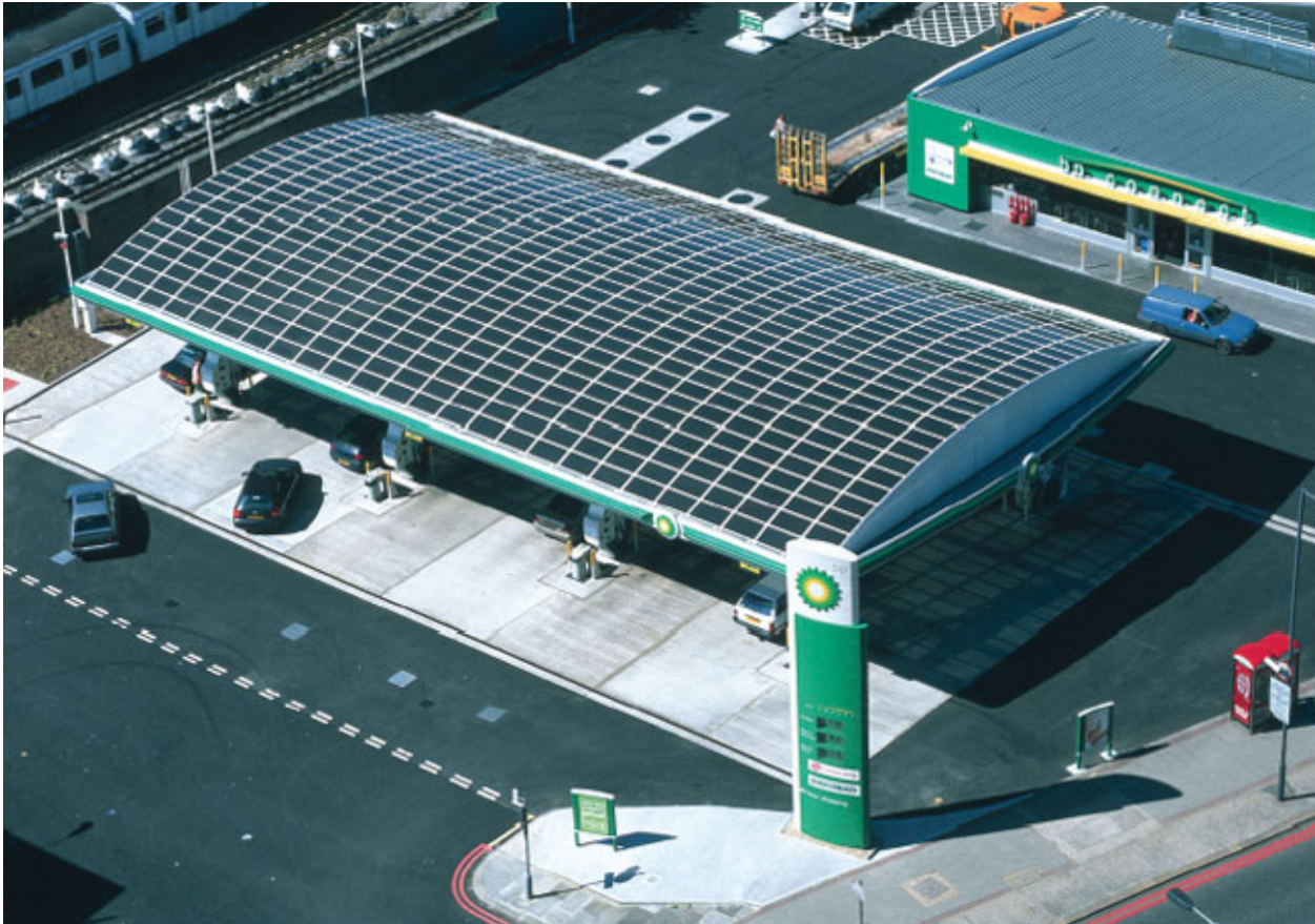
Figure 1.8 The roof of this petrol station in London has a large array of solar cells that convert solar radiation directly into electricity. This provides enough electricity to power the petrol pumps and lights.
