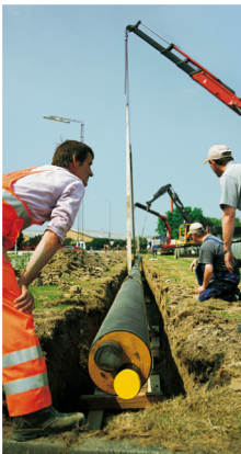
Figure 36 District heating pipes being laid. The flow and return pipes are surrounded with insulation and encased in a single pipe outer casing
