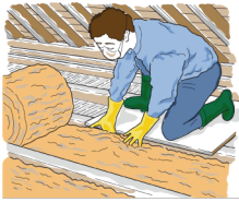
Figure 11 Rolling out a loft insulation base layer between the ceiling joists
