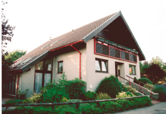
Figure 8 A polystyrene house. Despite its solid appearance, this house – built in Milton Keynes in 1986 – used a basic framework of insulating polystyrene blockwork into which concrete was poured. A brick skin was then added on the outside and the inside was plastered.
