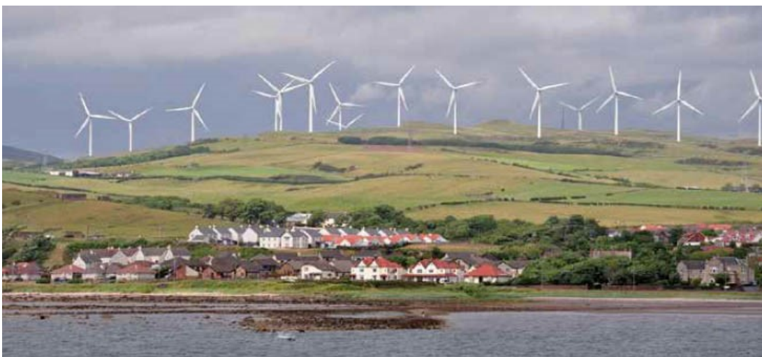
Figure 23 Ardrossan Wind Farm, Scotland, completed in 2004, is equipped with 2 MW turbines
