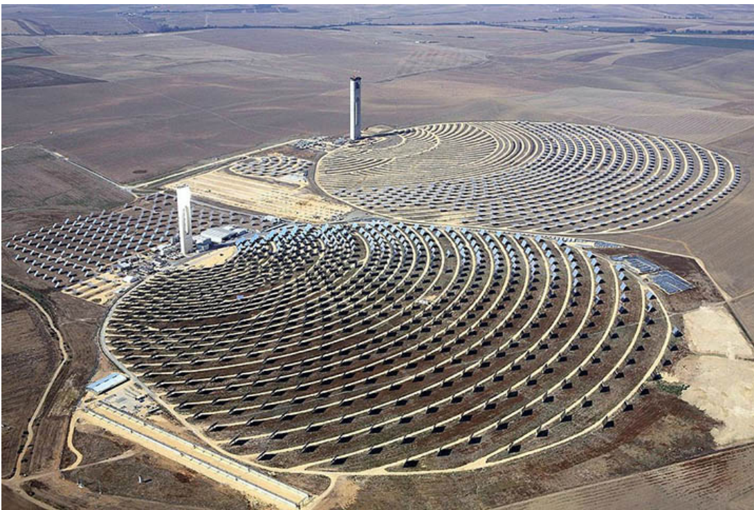
Figure 22 The Andasol PS10 and PS20 CSP systems near Seville, Spain. Installed between 2009 and 2011, they have generating capacities of 10 MW and 20 MW, respectively
