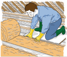
Figure 18 Rolling out a loft insulation base layer between the ceiling joists
