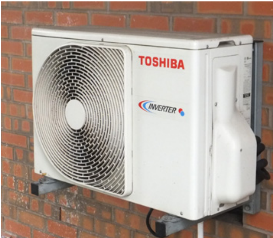
Figure 19 A fan-coil evaporator unit for an air source heat pump
