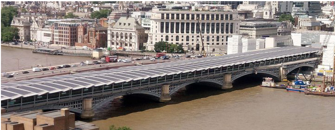
Figure 20 London's Blackfriars railway station has 6000 square metres of PV panels on its roof, supplying roughly a half of its electricity demand.
