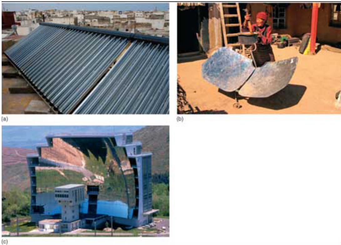
Figure 4 Types of solar collector. (a) Passive solar energy collectors mounted on the roof of an eco-hotel in Essaouira, Morocco. The hot water obtained from this system is also used in the local hammam , or Turkish bath. (b) A solar cooker based on mirrored plates arranged in the rough form of a parabolic mirror. The point of focus is the base of the pot, and little heating occurs away from that, so such cookers are safe to use. (c) Experimental solar furnace in the French Pyrenees.
