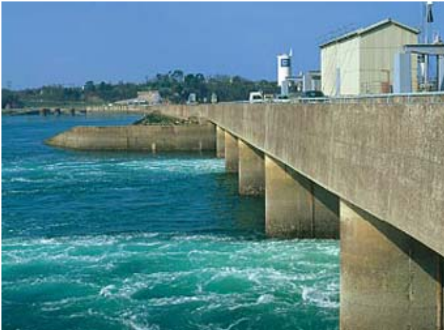
Figure 37: The 240 MW tidal barrage installed at the Rance Estuary in France
