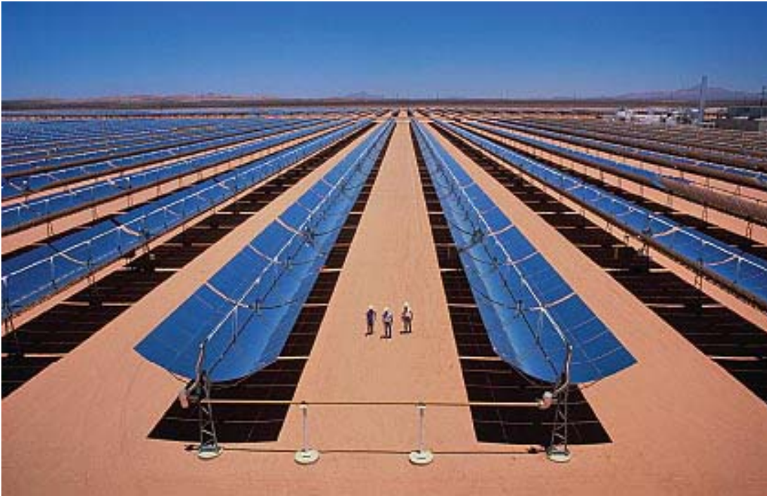
Figure 30: The largest 'solar thermal-electric' installation of its kind in the world, the Luz project in California's Mojave Desert, has a peak output of some 350 MW and occupies several square kilometres of land
