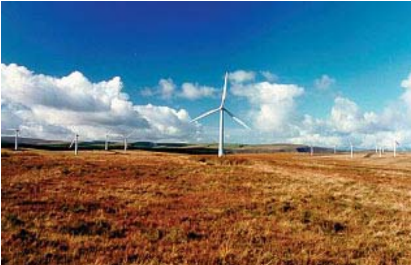
Figure 32: This wind farm, at Carno in mid-Wales, is one of the largest in Europe. It incorporates 56 wind turbines, each with a rotor diameter of 44 metres and a tower height of 31.5 metres. The total installed capacity is 33.6 MW, sufficient to provide power for some 25,000 homes
