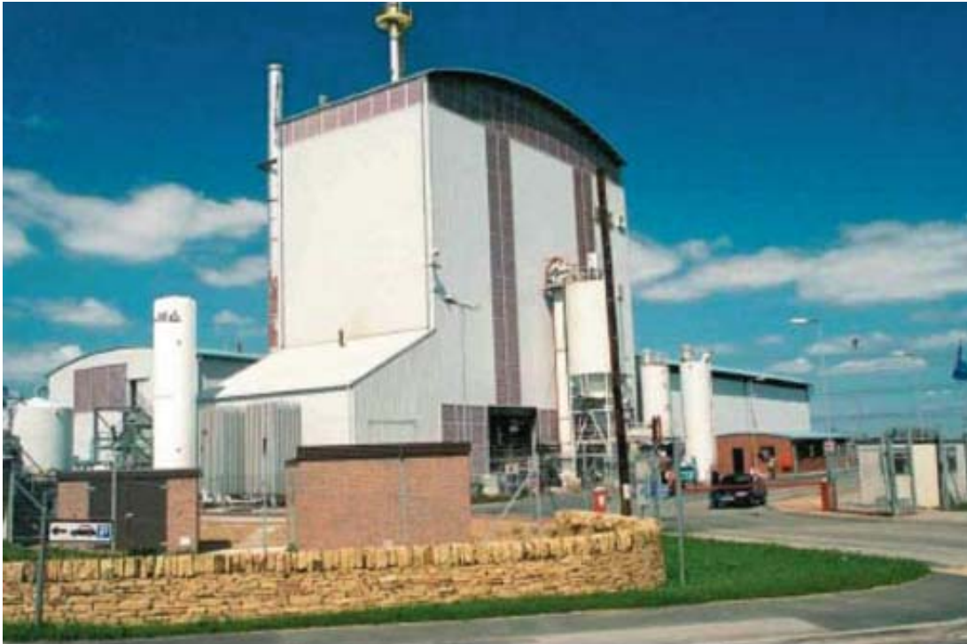
Figure 24: The 'Arbre' power station at Eggborough, Yorkshire, UK. Fuelled by wood chips, it has an electrical generating capacity of 10 MW
