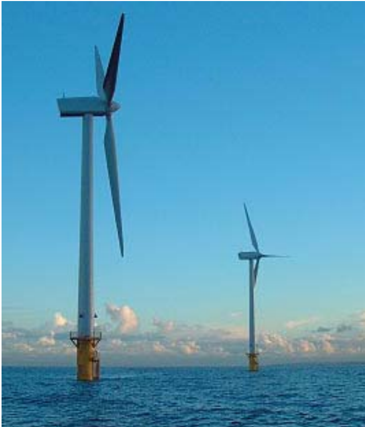
Figure 34: Britain's first offshore wind turbines, located 1 km away from the coast at Blyth harbour, Northumberland. The twin 2 MW turbines were installed in 2000 by a consortium including AMEC, Border Wind, Shell Renewables and the Dutch electricity utility Nuon
