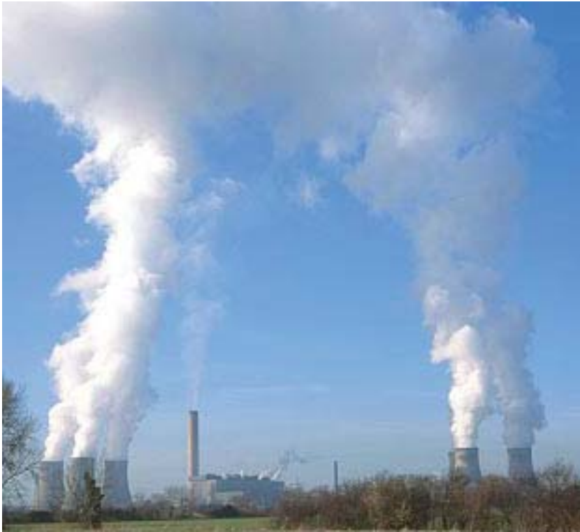
Figure 45: This coal-fired power station at Didcot, Oxfordshire, UK, was commissioned in 1972 and has a capacity of 2000 MW. Two-thirds of the energy content of the fuel burned in such power stations is dissipated by the cooling towers to the atmosphere in the form of steam
