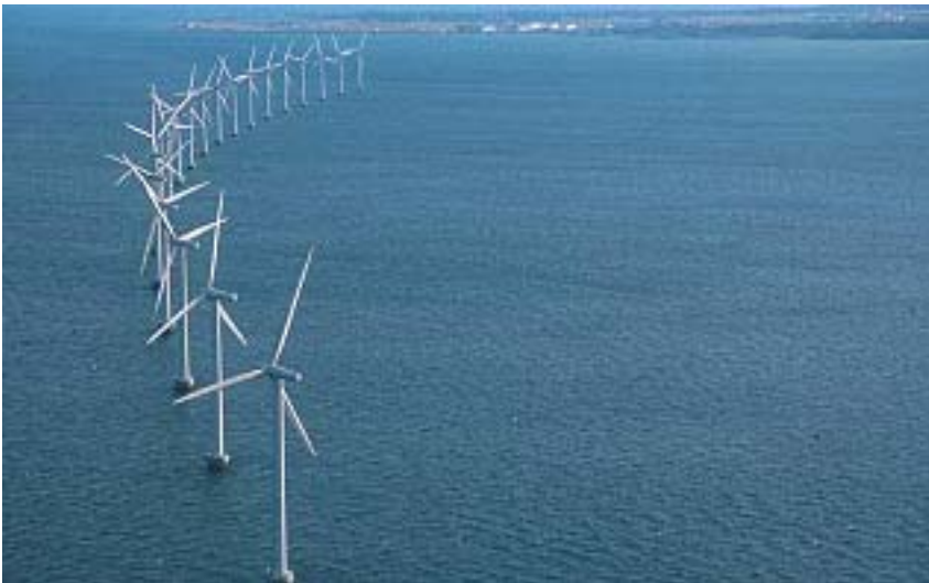
Figure 33: The Middelgrunden wind farm, completed in 2001, is located in the sea just off Copenhagen harbour in Denmark. It includes 20 two megawatt wind turbines, which provide 3 per cent of the electricity consumption of the Copenhagen municipality
