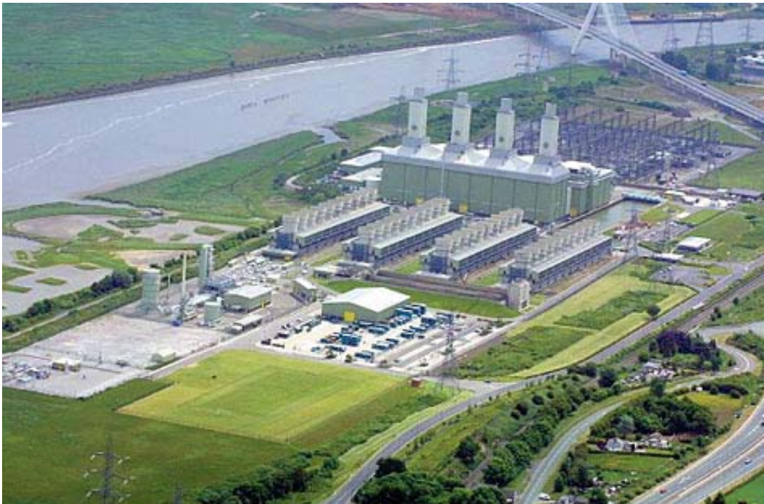
Figure 44: This combined-cycle gas turbine power station at Deeside in the UK was commissioned in 1994 and has an output of 500 MW
