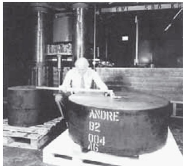
Figure C3 Bearing for a building in earthquake-prone regions
