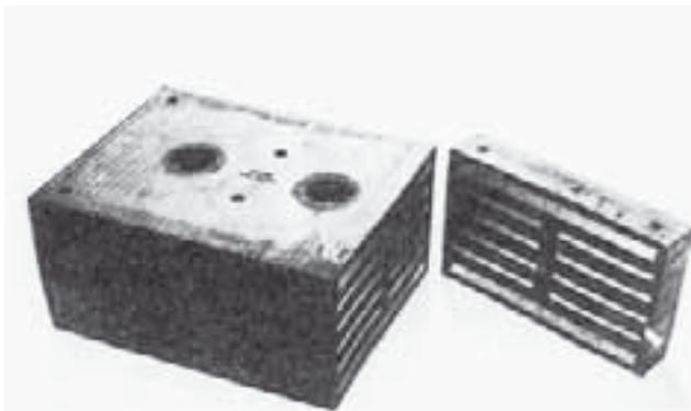
Figure C1 Typical bridge bearing
