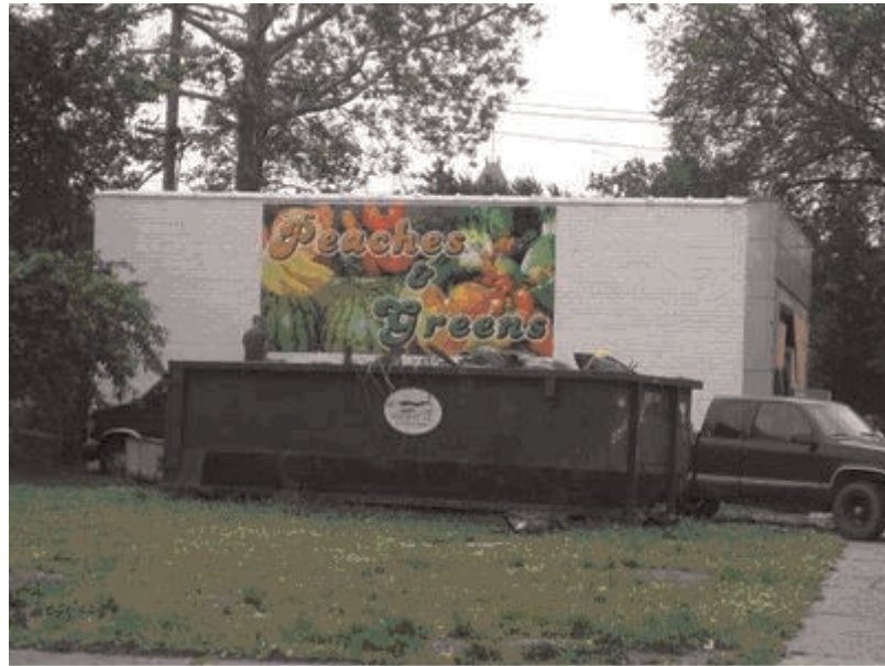
Side of the building – it used to be a dry cleaner (© Rachel C. Parton)
