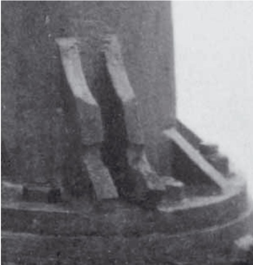
*Figure C16* Fractured lug on pier 3
