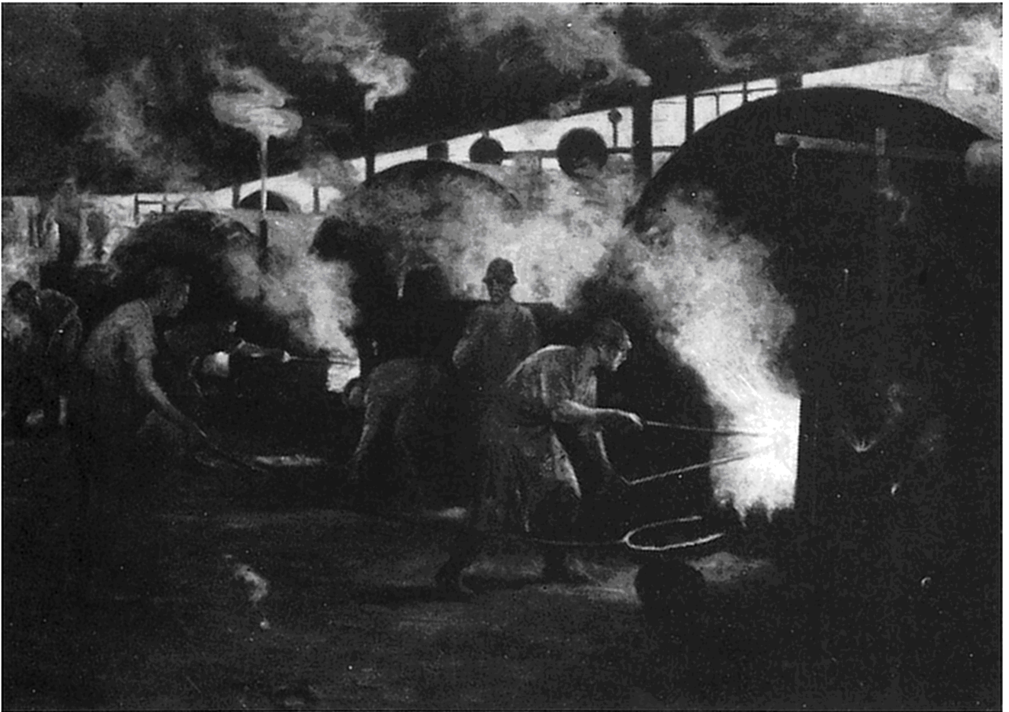
The Puddling Furnace, Cwmbran Ironworks, from the original oil painting in the Department of Industry, National Museum of Wales
