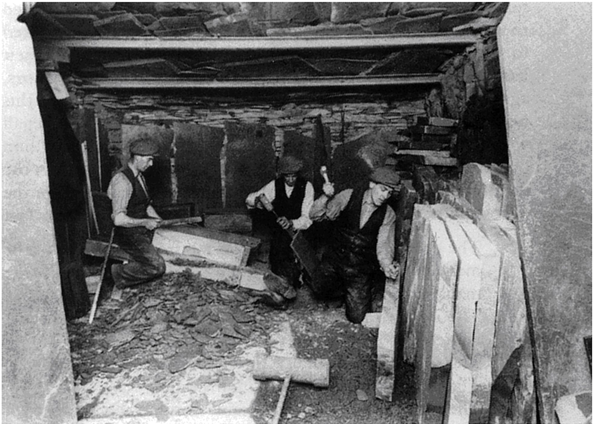
Slate splitting, Dinorwig Quarries, c. 1910
