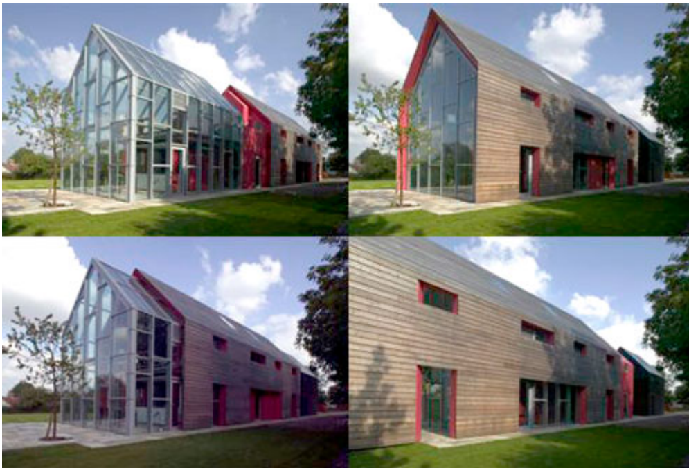
Figure 9 dRMM's Sliding House has mobile walls and a roof that glides along rails to
