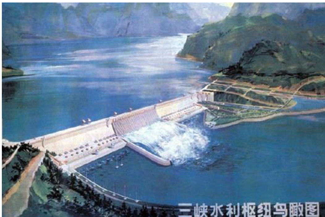
Figure 18 The Three Gorges dam in the Yangtze in China is one mile long and 181 metres high, with an installed generating capacity of 18,000 Megawatts.
