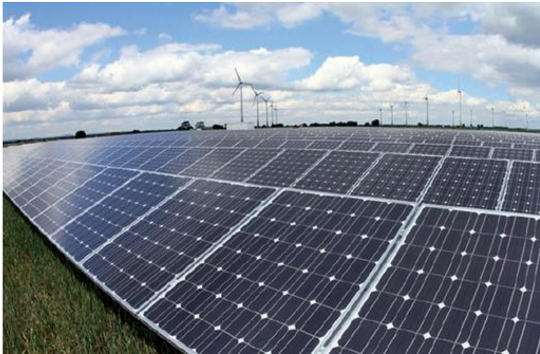
Figure 10 This 1 MW ‘sun farm’ in Lincolnshire, UK, is adjacent to a wind farm, with the aim of enabling the higher electricity contribution from wind in winter to compensate for lower electricity output from PV, and vice versa in summer (source: Ecotricity)
