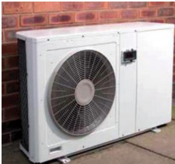
Figure 19 Fan-coil unit for an air-source heat pump
