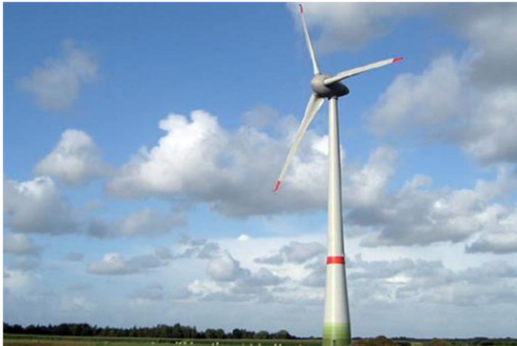
Figure 21 E126 7.5MW 126m diameter wind turbine, an example of a very large turbine (source: Enercon, 2011)
