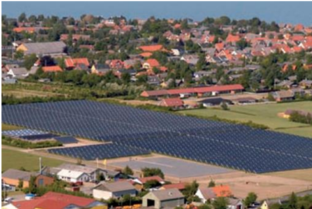
Figure 17 An 18 000 m 2 array of collectors feeding a district heating system at Marstal in Denmark
