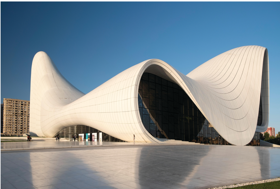
Figure 3 The complex curves of Zaha Hadid Architects' Heydar Aliyev Center in Azerbaijan were only possible using algorithmic tools
