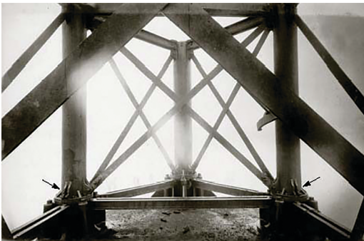
Figure 28 Remains of pier 3, looking west. The broken east-facing lugs are indicated by the arrows
