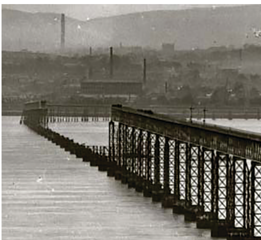
Figure 21 The missing high girders section, looking north, with Dundee in the background. Note the many tall chimneys, which were clearly unaffected by the storm. The photograph also shows the steep downward gradient of the final part of the bridge
