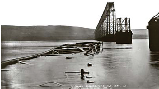
Figure 22 Remains of the high girders lying on the estuary floor, with the south side of the fallen bridge in the background
