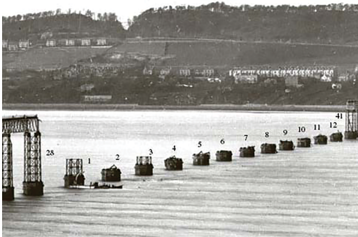
Figure 20 Fallen piers as seen from the south bank of the firth. For the purposes of the BoT investigation, the piers between 28 and 41 were numbered 1–12, as shown in the picture
