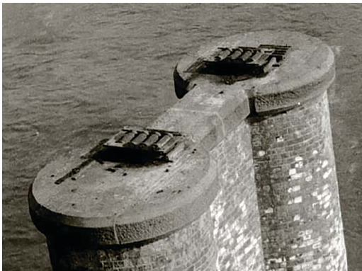
Figure 37 Top of one of the brick piers of the old Tay bridge showing the cast-iron roller bearings in situ before the pier was demolished
