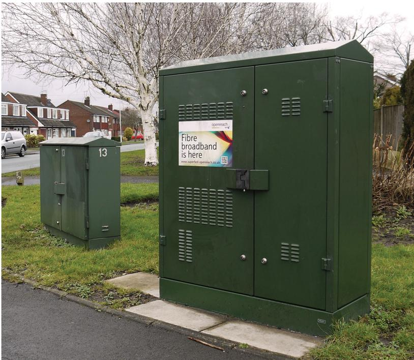
**Figure 4.7** Fibre box used with VDSL2
