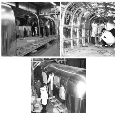
Three views of the first Mobile Quarantine Facility under construction at Airstream's Jackson Center, Ohio, plant. Image credits: courtesy The Airstream Company.
