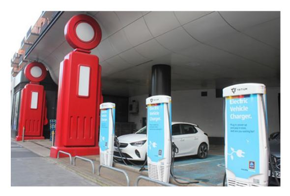
Figure 14: Three 50 kW rapid BEV chargers in a repurposed petrol station forecourt in London.
