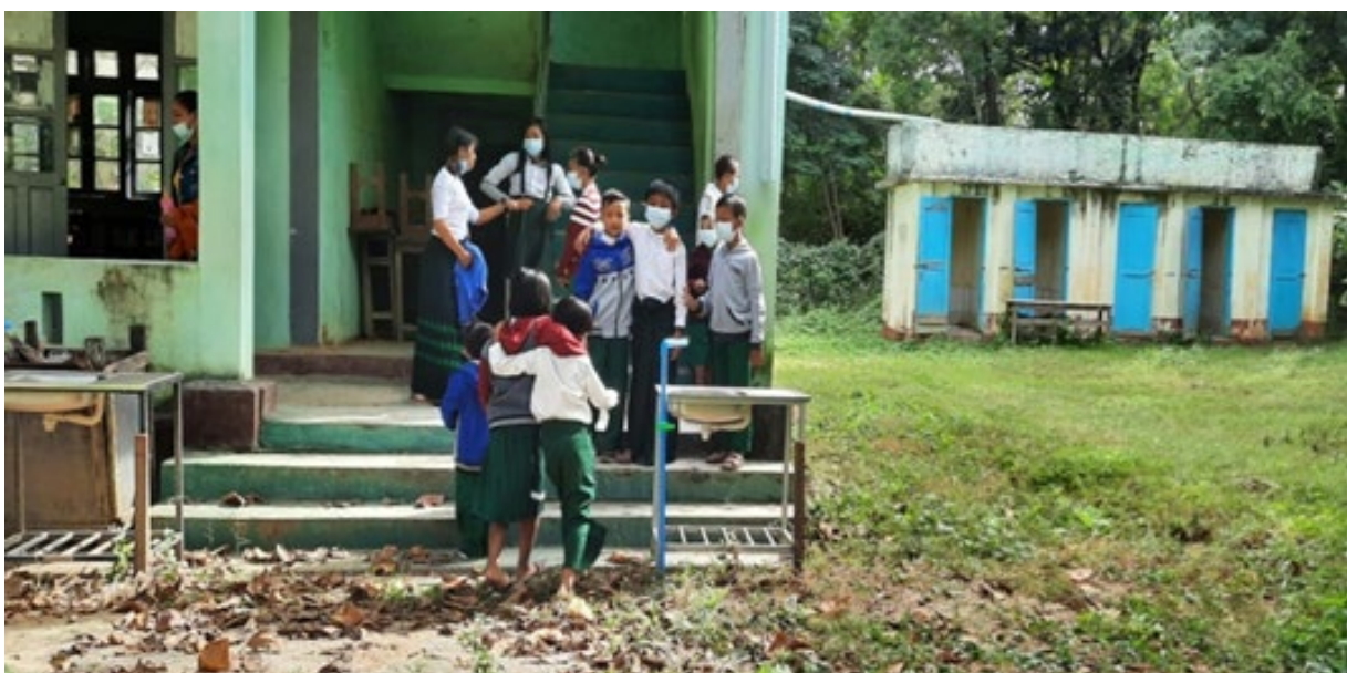
Figure 6.4 School latrines and handwashing facilities
