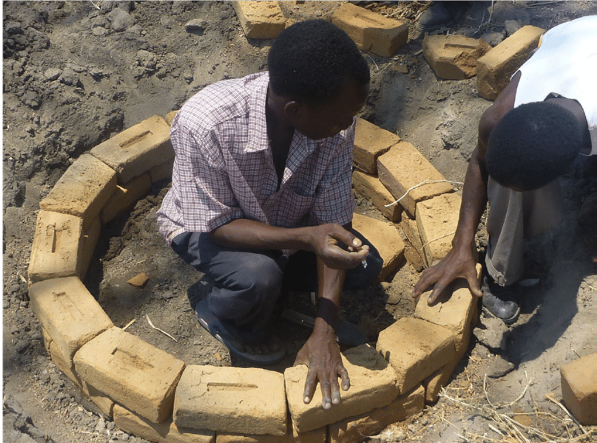
Figure 5.3 Innovative non-cement designs for pit latrines in difficult contexts caused by soil conditions. Developed by teams of community members in a participatory design process organised by UNICEF Malawi.
