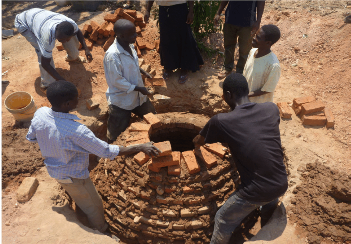
Figure 5.3 Innovative non-cement designs for pit latrines in difficult contexts caused by soil conditions. Developed by teams of community members in a participatory design process organised by UNICEF Malawi.
