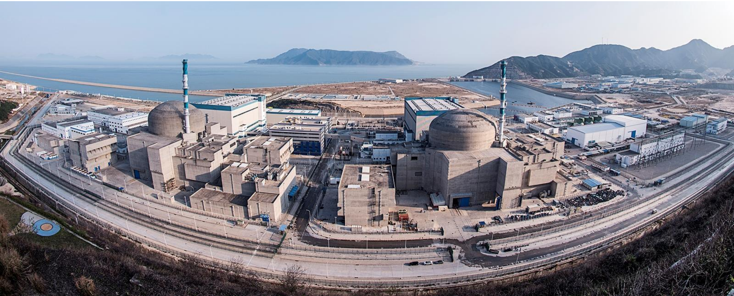
Taishan Nuclear Power Plant, Units 1 & 2, Guangdong, China
