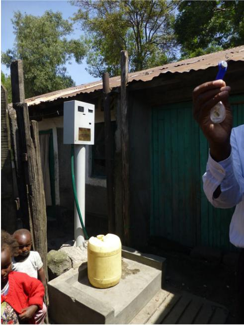
*Figure 13.5 A prepaid water meter. The man standing to the right is holding the small blue credit token that is inserted into the meter to obtain water.*
