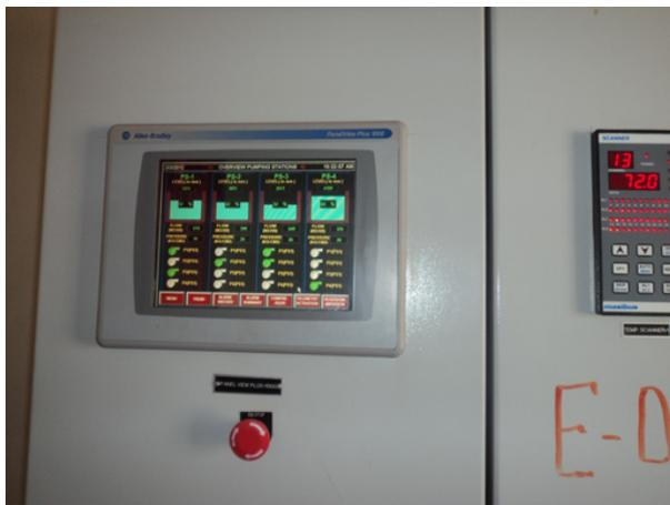
Figure 6.3 Control panel in a water treatment plant.
