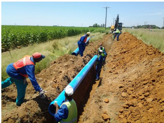
Figure 7.2 Plastic water mains being laid.
