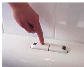
*Figure 11.4 The buttons on a dual-flush toilet cistern.*
