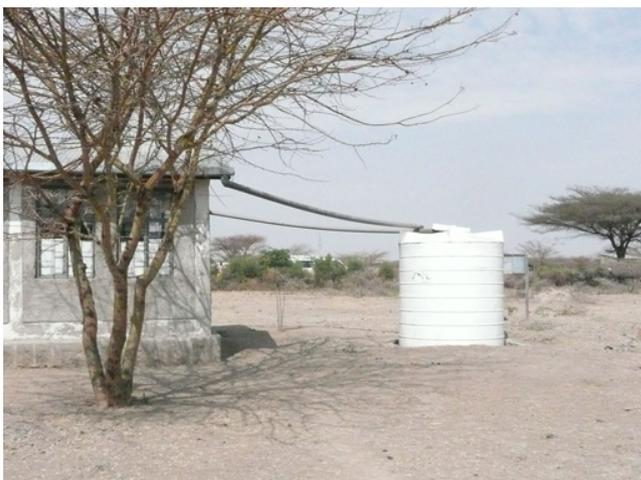
*Figure 3.13 Rainwater is collected from the roof of this rural health post and stored in a covered, watertight cistern.*
