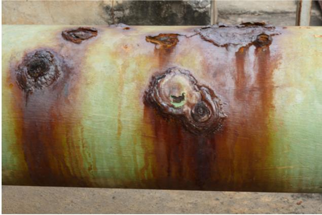
*Figure 7.4 A section of corroded water pipe.*
