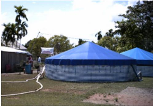
Figure 14.8 Emergency water treatment tanks.
