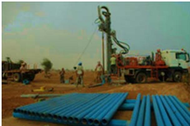
Figure 3.8 Drilling rig for a borehole.
