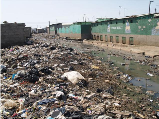
*Figure 1.4 Accumulated solid waste and effluent from a latrine block have filled a drainage canal in Accra, Ghana.*
