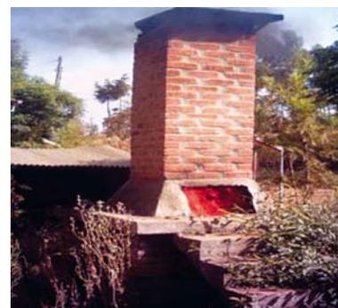
Figure 7.3: An incinerator used for burning healthcare waste. (Photo: Muluken Azage)
