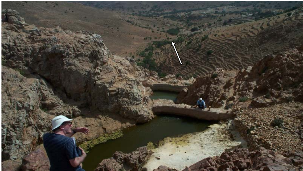
Figure 7.4: Local reservoirs “le petit barrage”. The arrow points to where water is collected from at the bottom of the mountain during drought years (Source H Moore).
