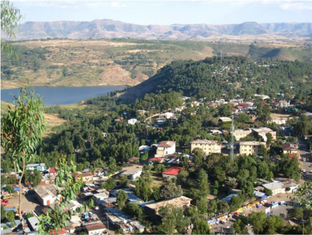
Figure 3.12 Gondar's water supply comes from the Angareb reservoir, which was created by damming the river.
