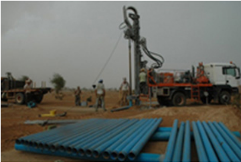
Figure 3.8 Drilling rig for a borehole.
