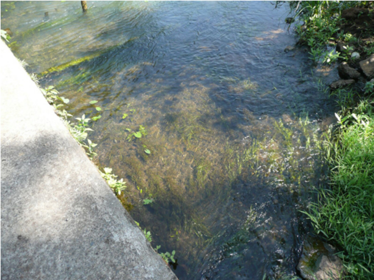
Figure 3.11 Protected spring providing water for Bahir Dar. The concrete slab on the left covers and protects the source of the water.
