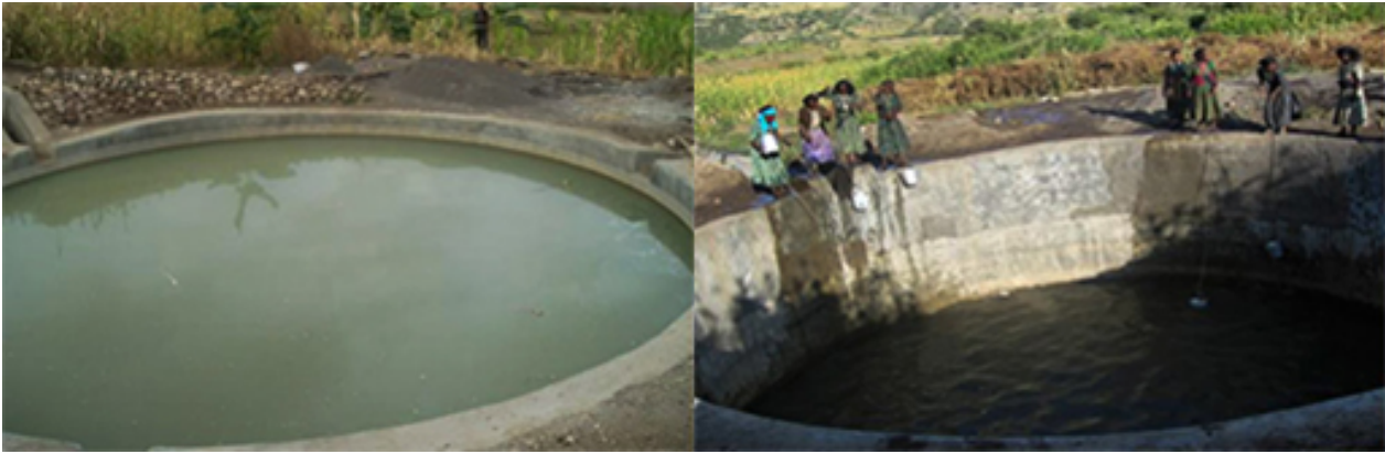
Figure 3.14 Rainwater storage ponds in Amhara Region.
