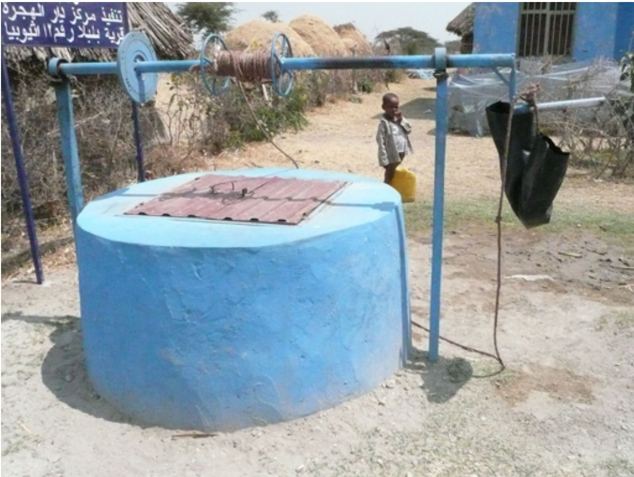
Figure 3.5 Protected well with concrete surround and a lid. Note the black plastic bucket is suspended off the ground to keep it clean.
