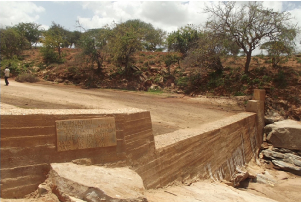
Figure 3.15 A sand dam in Kenya.
