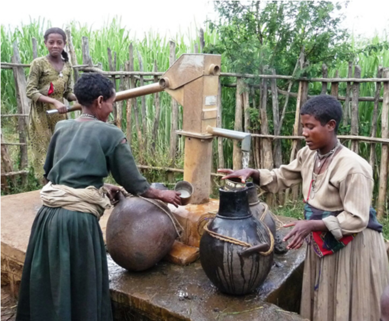
Figure 3.6 Hand pump over a protected dug well. Note the concrete surround and the fence to keep out animals.
